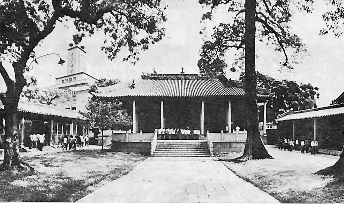
The house where the National Institute of the Peasant Movement was.
